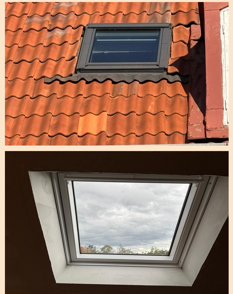
Skylight window after replacement
