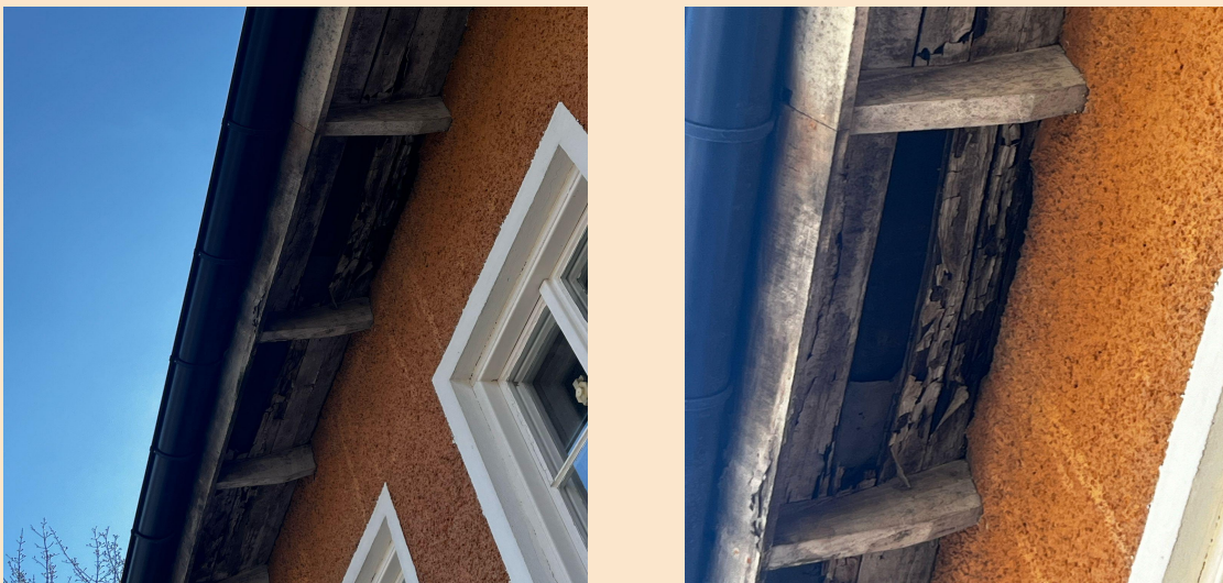
Rotten roof before
